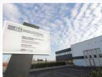
Latisana – ITALY. Production Plant.
